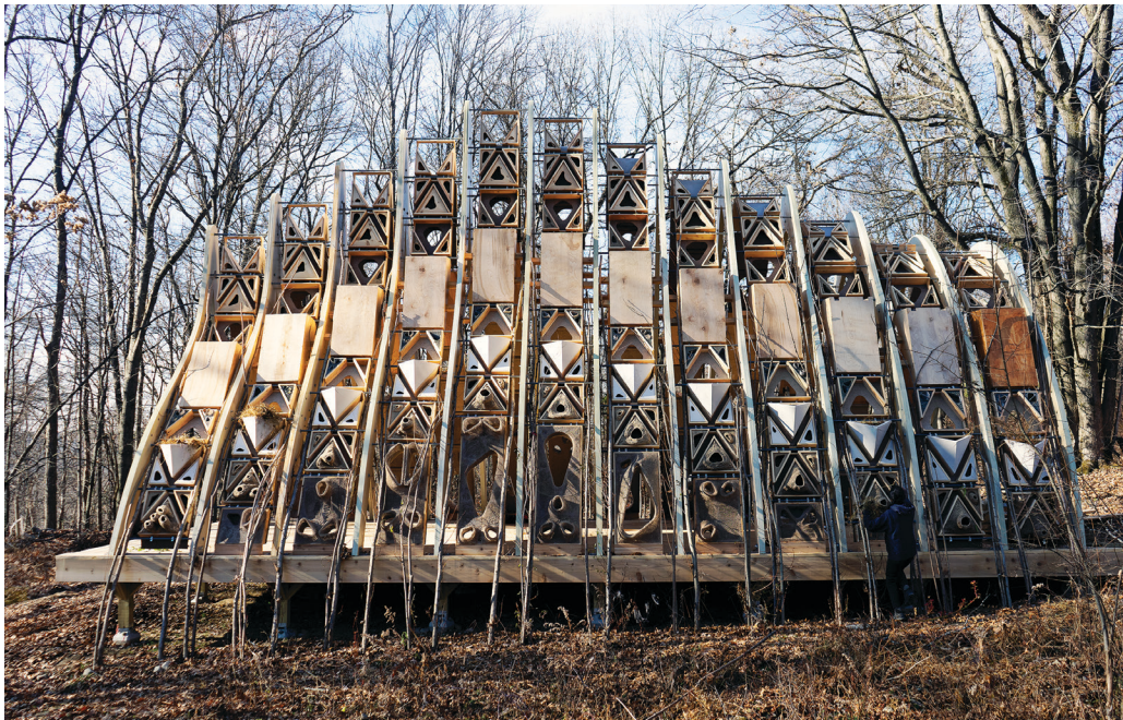
Terreform ONE, Fab Tree Hab, New Windsor, New York, December 2023 (bottom) and June 2024 (top). The structural scaffolding and live plant grafting for the Fab Tree Hab “terrestrial reef” phase were completed in early December 2023. The living structure will continue to grow and mature over the next decade. Photos courtesy the architects.
